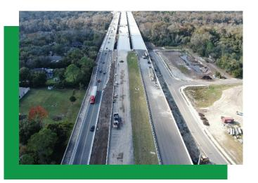
One of the parkway's signature features is being built along Section 6 – a new, much higher Wekiva River crossing with enhanced aesthetics. The three, 60-foot-tall bridges put the deck in the tree canopy to visually buffer it from surrounding communities. The higher crossings will open the river for an enhanced user experience by kayakers and canoeists. Animals will be able to pass safely underneath along the riversides, as opposed to having to cross S.R. 46.
